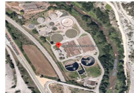
SMARTech2b and Downstream SMARTech B - Manresa WWTP (Spain)
